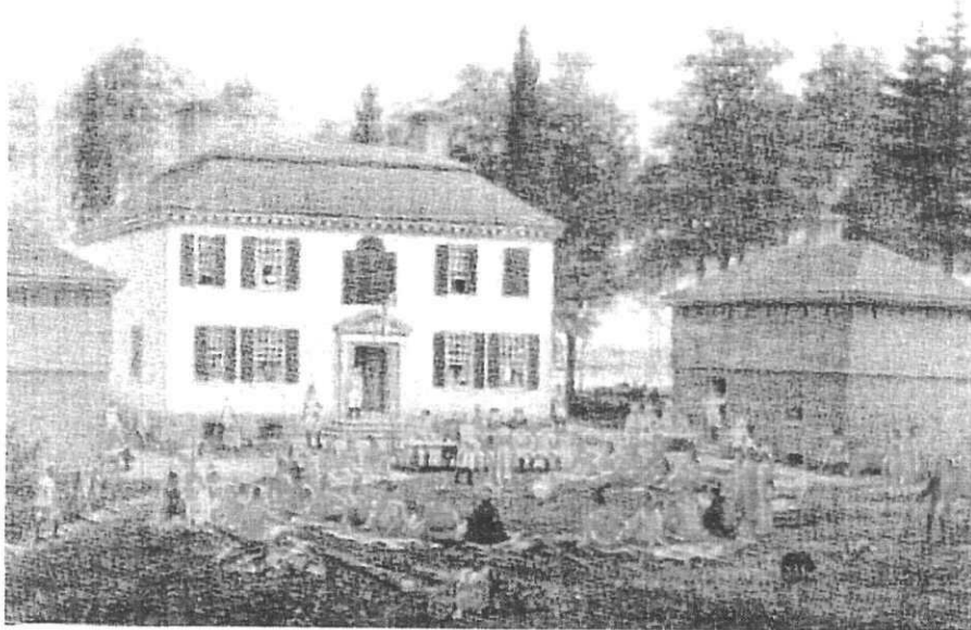
"The Council Fire at Johnson Hall"
